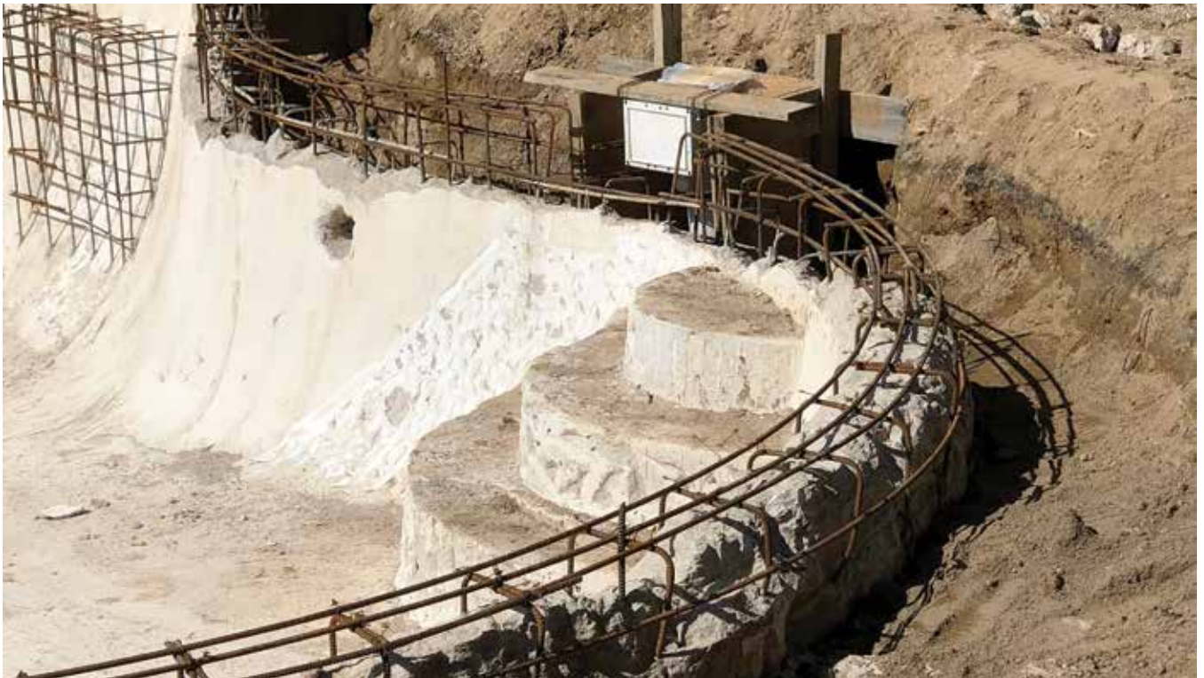
Fig. 1: Close-up of raised bond beam with supplemental reinforcing and roughened substrate
