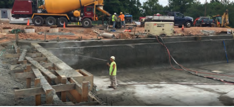
Wetting down freshly shot walls after finishing
